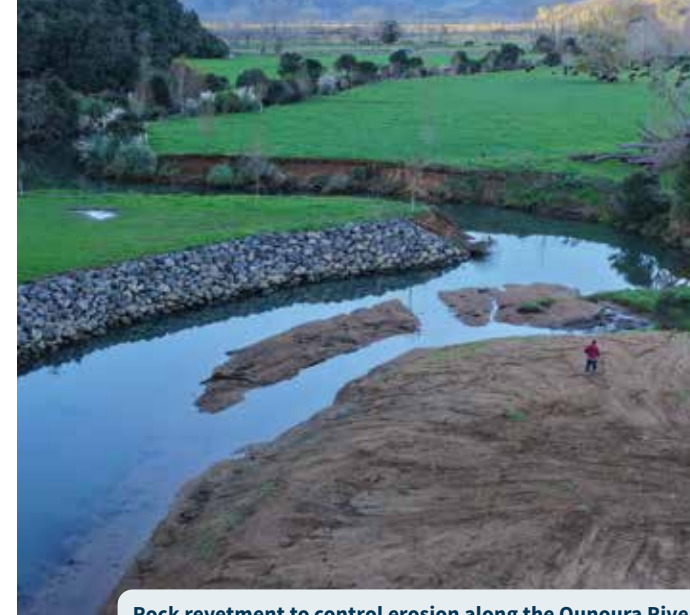
Rock revetment to control erosion along the Ounoura River.
