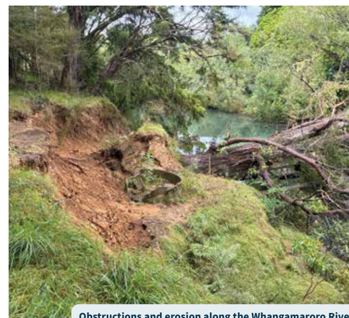
Obstructions and erosion along the Whangamaroro River.
