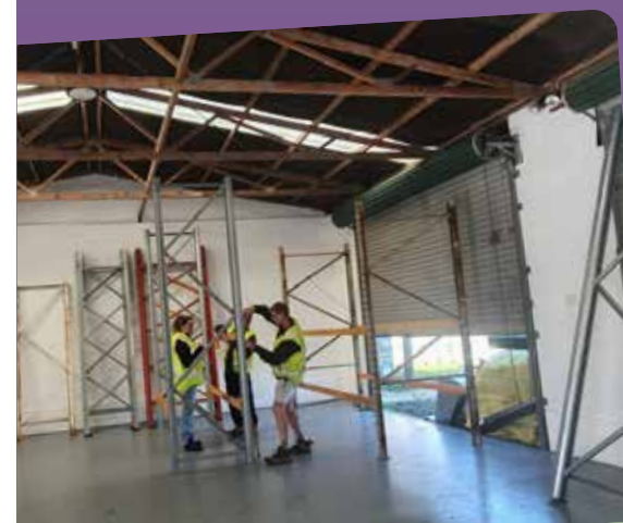
Setting up racking at Whitianga's resource recovery centre.
