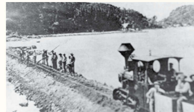
Whangapoua Harbour Kauri Freehold Gold Estates Tramway – ca 1865 – Kraus locomotive, 7.5 tons to haul 25 tons on a gradient of 1 to 25.
